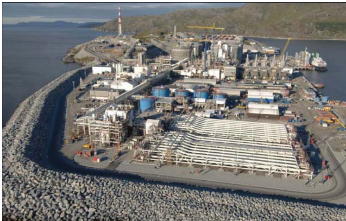
Space limitations on the slug-catcher dictated the "bent finger" design (Fig. 6; photo by Øyvind Hagen, Statoil).
