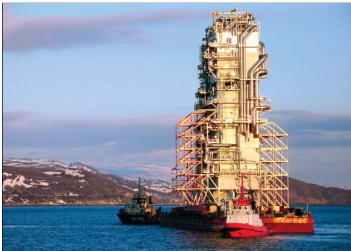
In July 2005, the cold-box assembly containing the three cold boxes supplied by Linde arrived at Melkøya (Fig. 7; photo from Linde AG)
